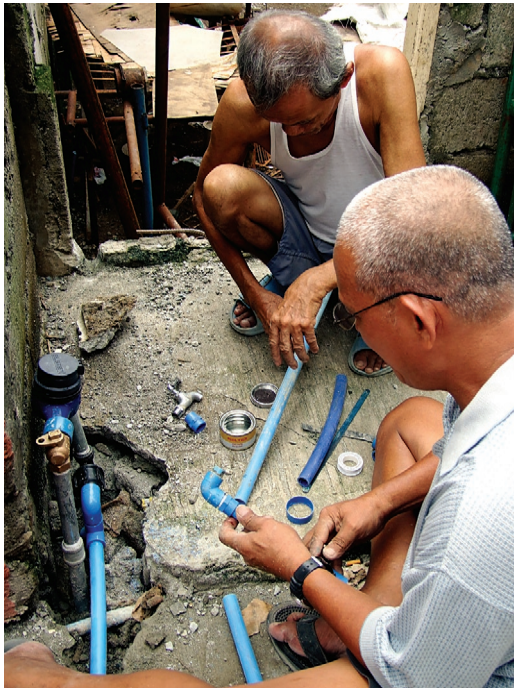
Installing metered pipelines in Manila's Alitaptap community
