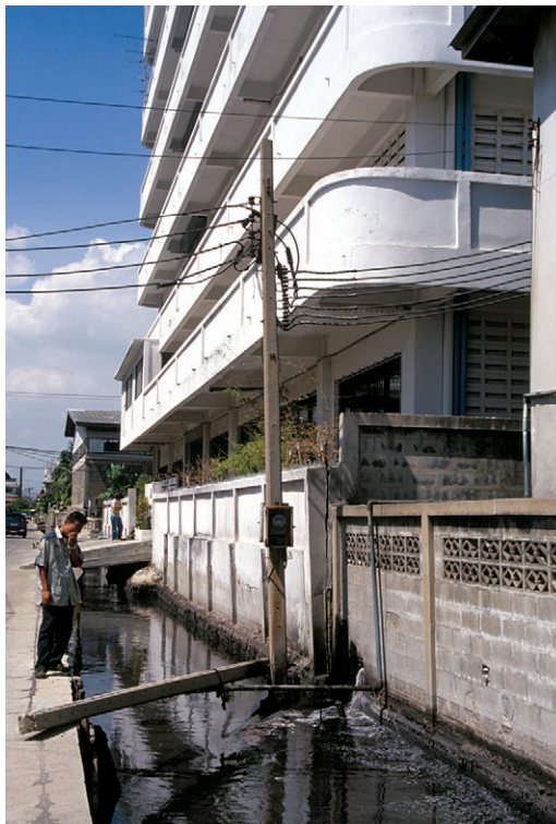
Urban sewage canal in Thailand
