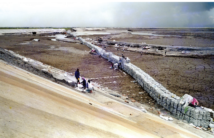
Mega Dike or the FVR dike in central Luzon being supported by sand bags.
