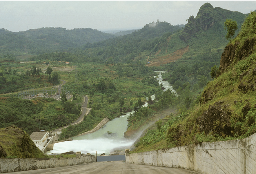
Hydro energy-generating dam, Indonesia
