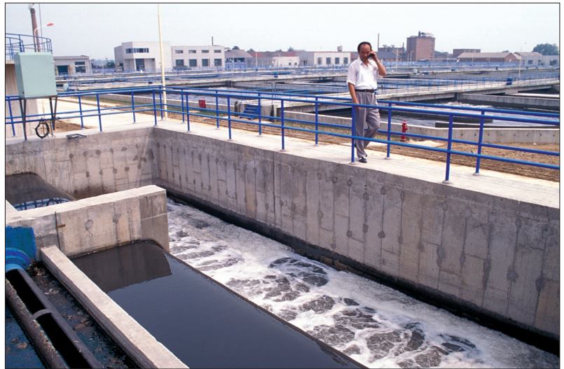
Inspecting Tangshan City Dongjiao Waterwaste Treatment Plant, People's Republic of China
